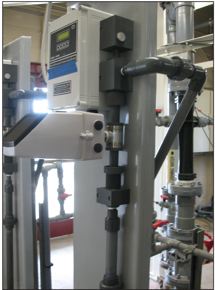
Each feeder automatically regulates in both fixed and variable control modes, including fixed feed rate, flow paced, residual control, and compound loop.
