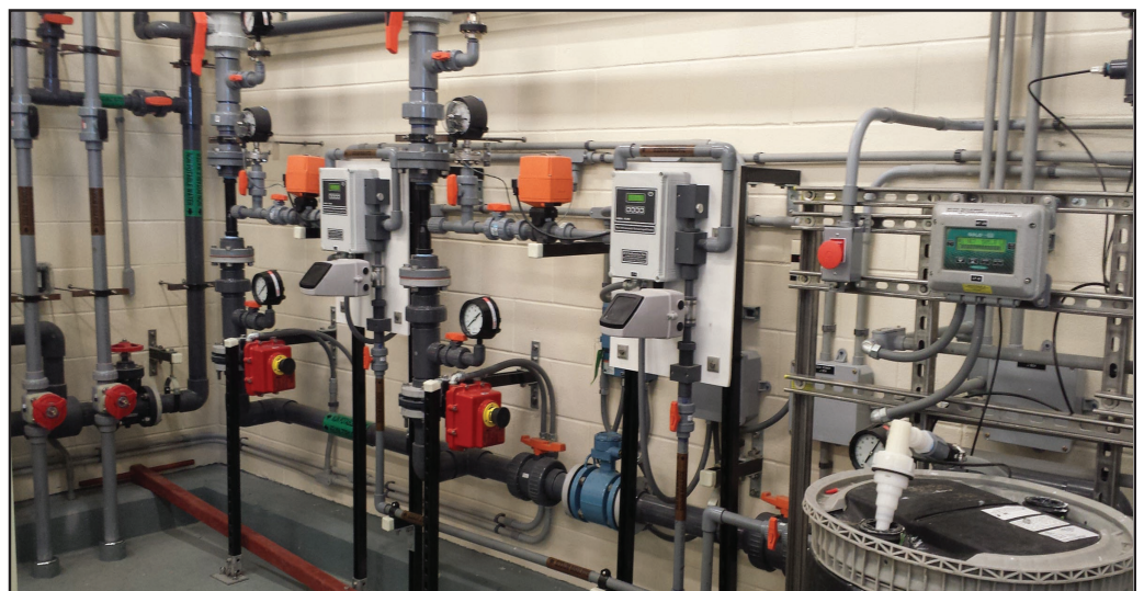
Patented vacuum chemical feeder system delivers sodium hypochlorite (NaOCl) for dechlorination, providing for disinfection of untreated discharges of combined sewer overflows (CSOs).
