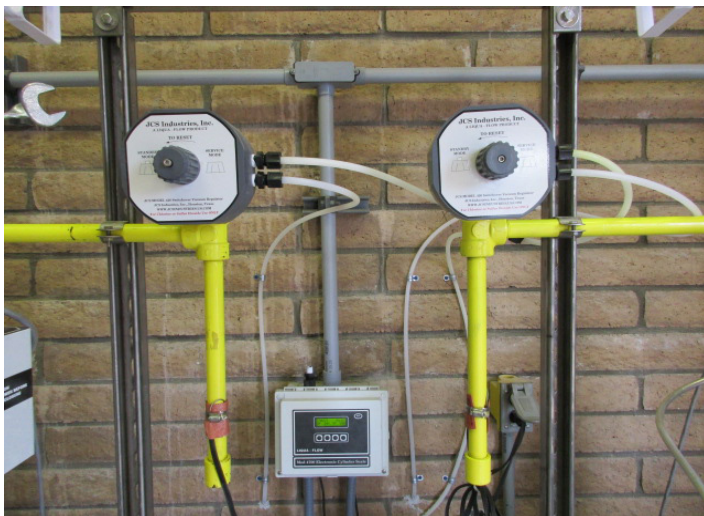
Automatic vacuum regulators, with switchover, have electric motors that rotate valve stems toward open or closed position for alignment, tests, and remote operation. There are no large signal cables.
