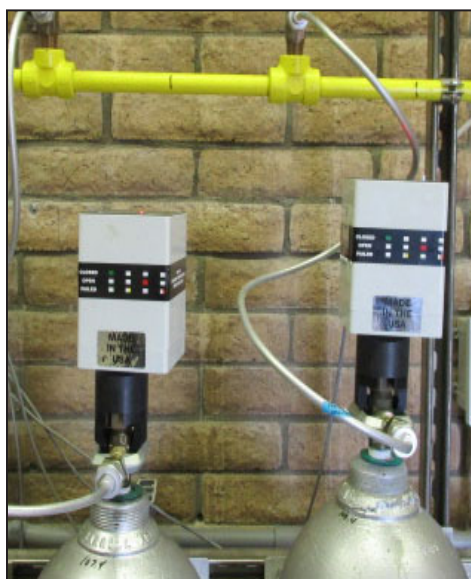
The JCS Robo-Control automatic shutoff system, left, is electrically operated, and provides for battery backup. It remotely closes valves, and mounts without interfering with other mounted hardware. The gas vacuum chemical feeder, right, includes a control module for complete electronic control and communications. Available control modes include flow proportional, residual, and compound loop.
