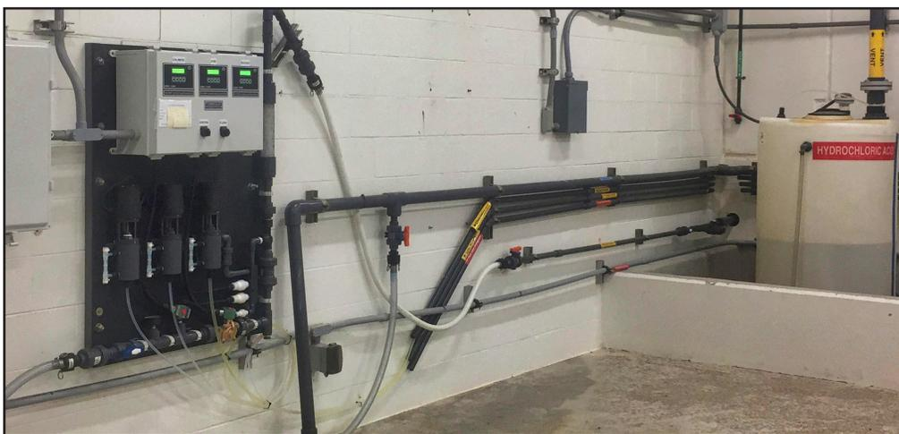
Switching to three-precursor vacuum generator-feed, from batch-generator-pumping, for introducing chlorine dioxide (ClO<sub>2</sub>), cut chemical costs, gained new management control for generation and feed equipment, and ended a pesky maintenance burden.
