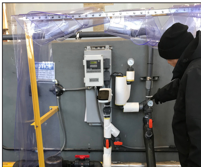
Still further application of advanced vacuum feeders, for caustic feed, is now being tested as further replacement for metering pumps.
