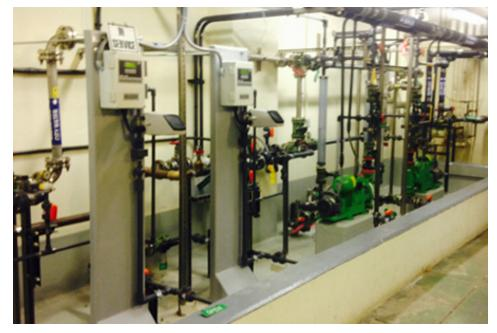
new water and wastewater plants. The capital investment in a vacuum system for a typical 1,000 GPD water system can be less than half of that for a metering pump system. Operating expenses in those cases are about a third of the cost because of the relatively high cost of maintenance kits and energy needed for metering pumps. Larger-capacity plants that would require big pumps can install liquid vacuum feeders in much less space.
